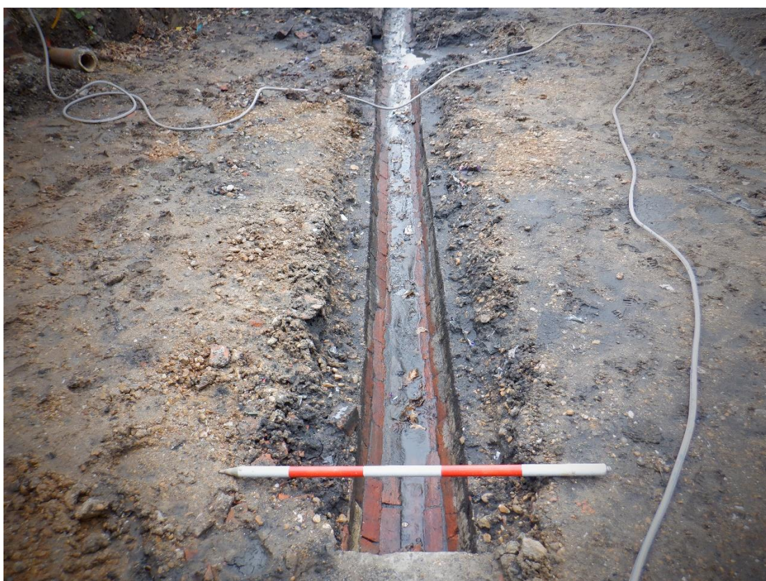
Plate 4. Exposed Victorian drain (looking East)
