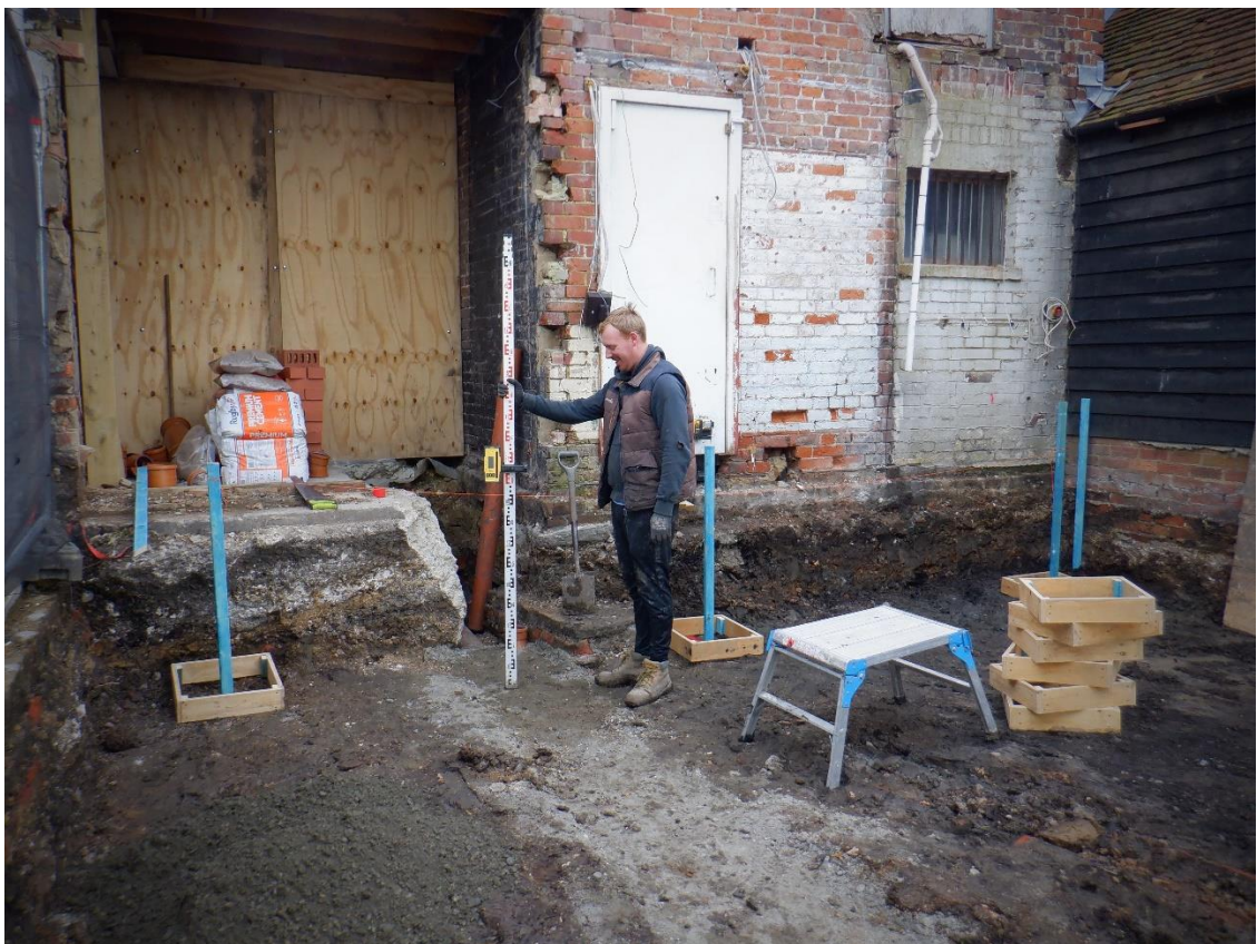
Plate 6. Completed site reduction (looking South-East)
