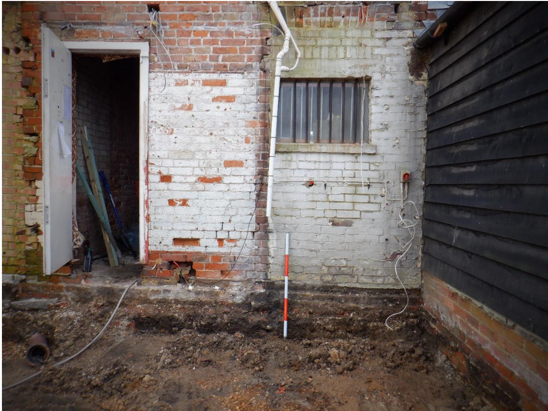
Plate 5. Completed site reduction (looking East)
