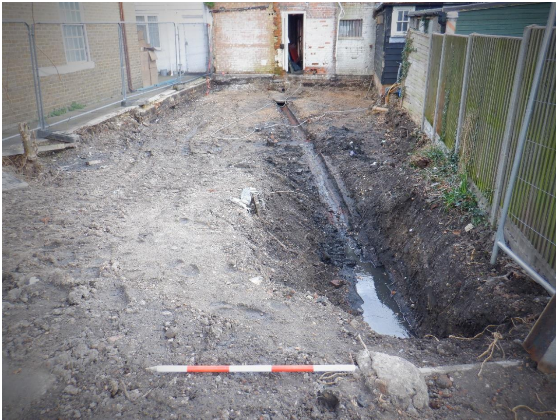
Plate 2. Ground reduction (looking East)
